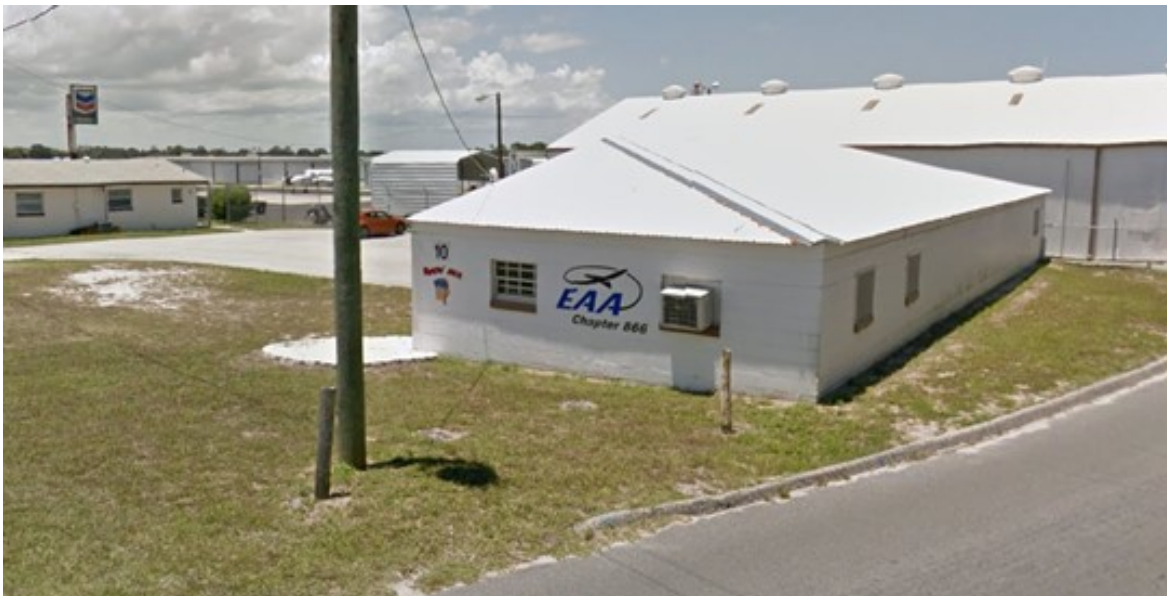
Building 10 at Arthur Dunn Airpark, Home of EAA Chapter 866
