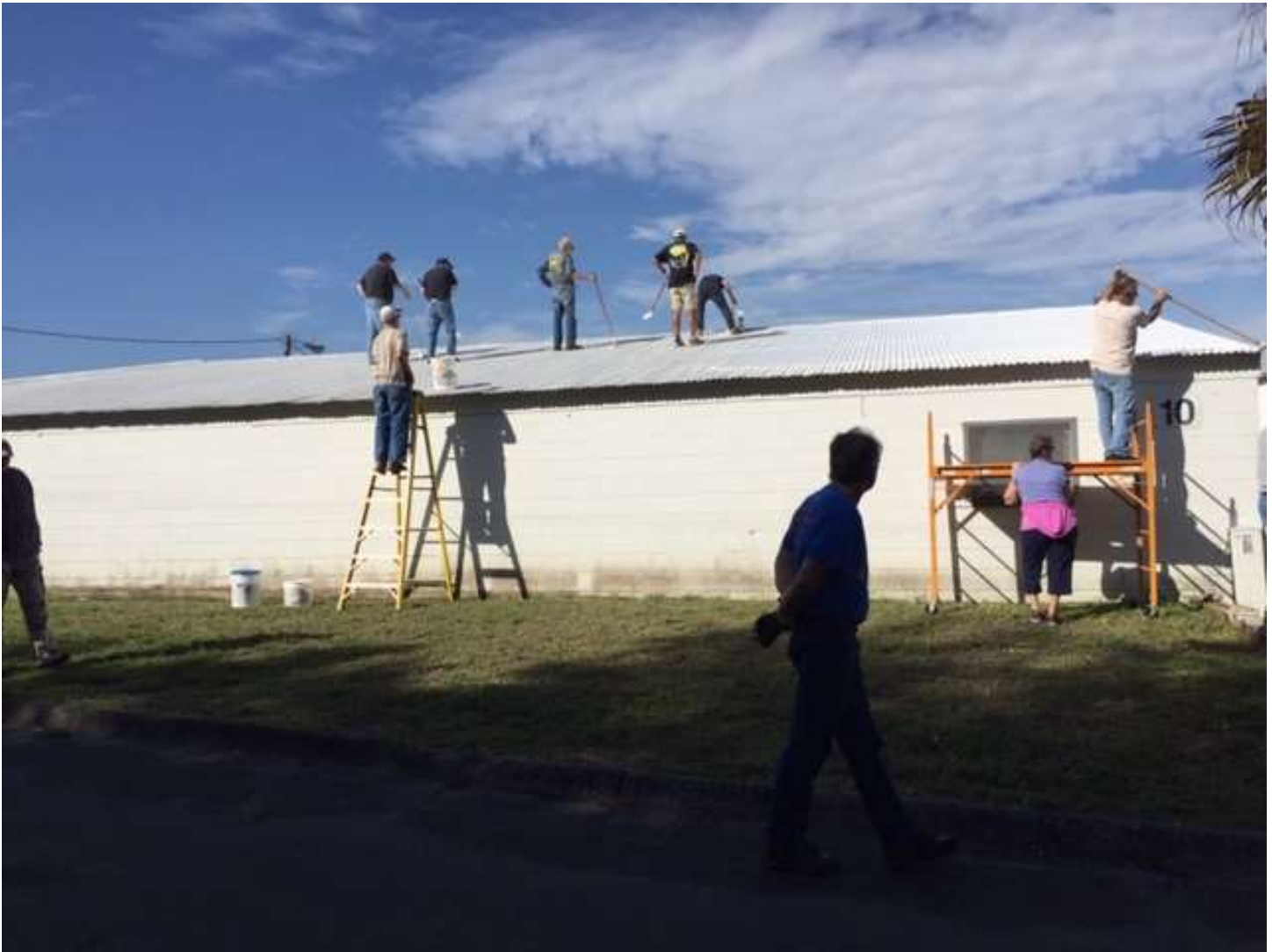
Work in progress – good crew, approaching halfway mark
