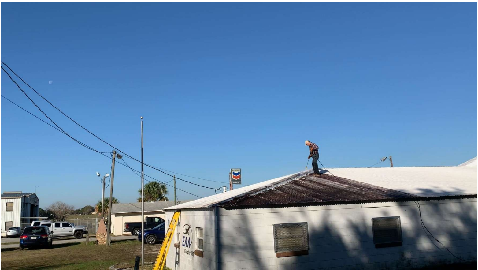
Bob Rychel pressure washing Bldg. 10, Jan 14, 2023
