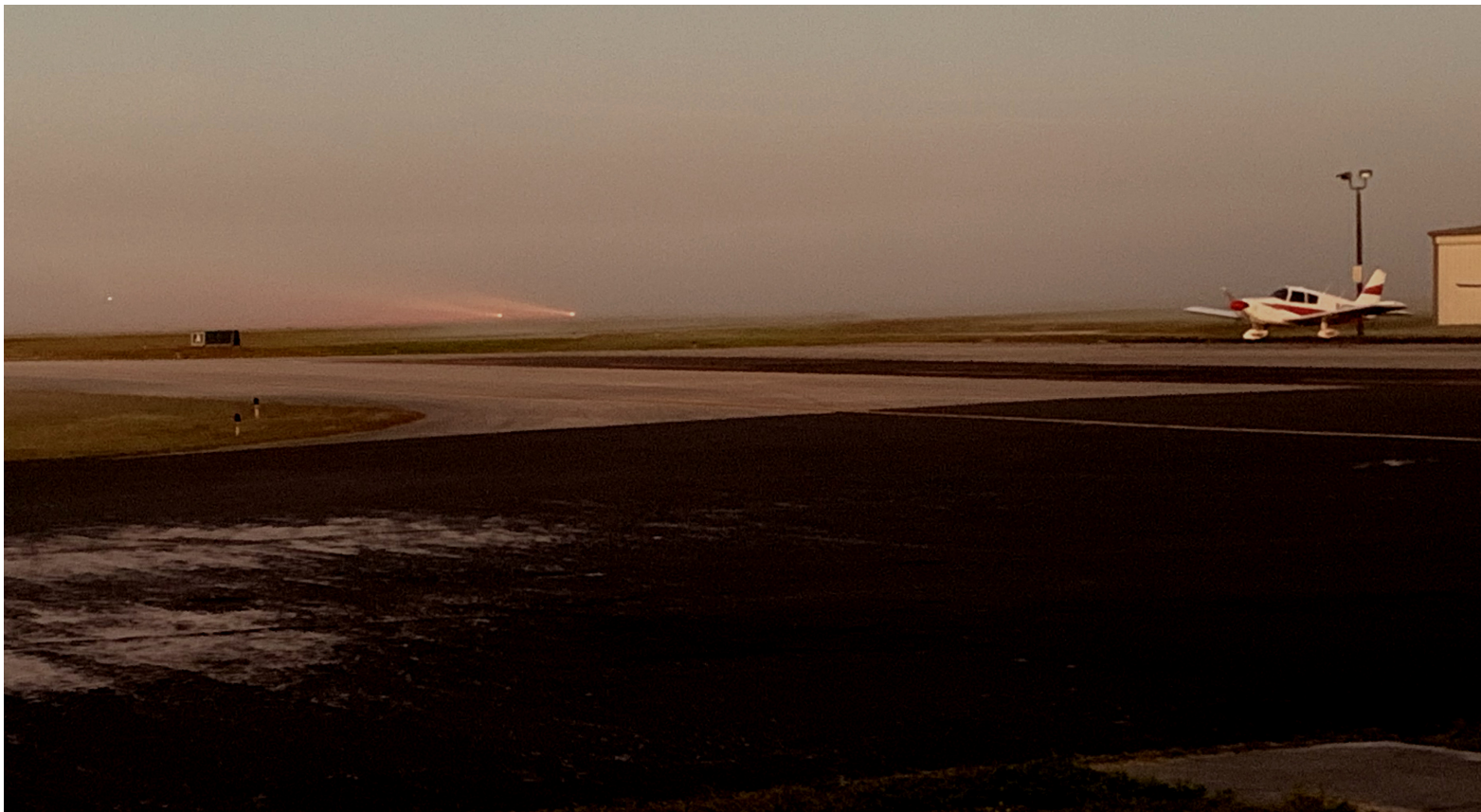
New PAPI installed and functional rwy 33 at Dunn
